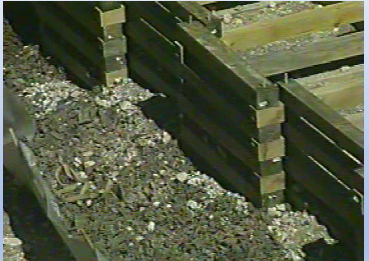
Timber Bin Wall with TDA Backfill, River Road, Arlington, VT
