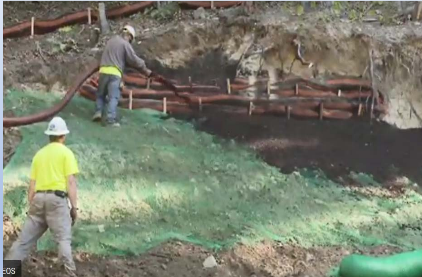
Compost socks and blankets installed post-Irene, Jamaica, VT
