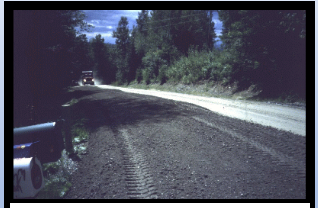
RAS/RAP/Gravel placement, Huntington, VT
